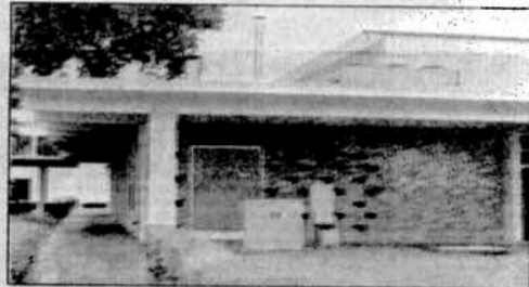
The Billy Harrison Health Building on the Gulf Coast campus. News Herald Photo: Terry Barner
